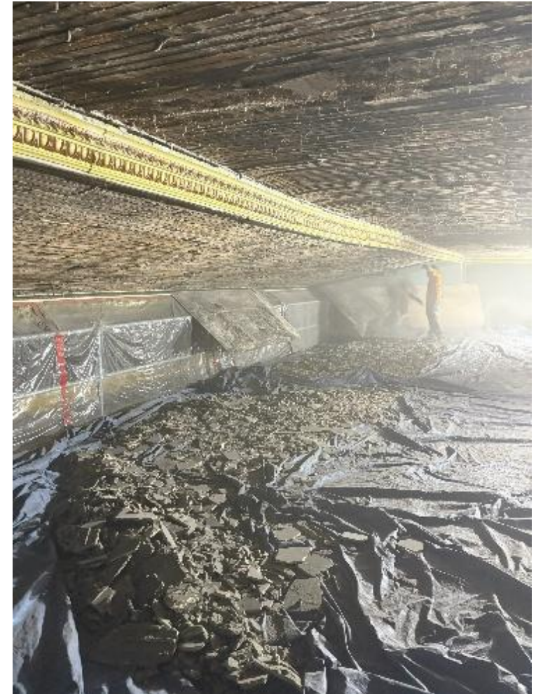
Plaster is down, to be soon out of the building.
