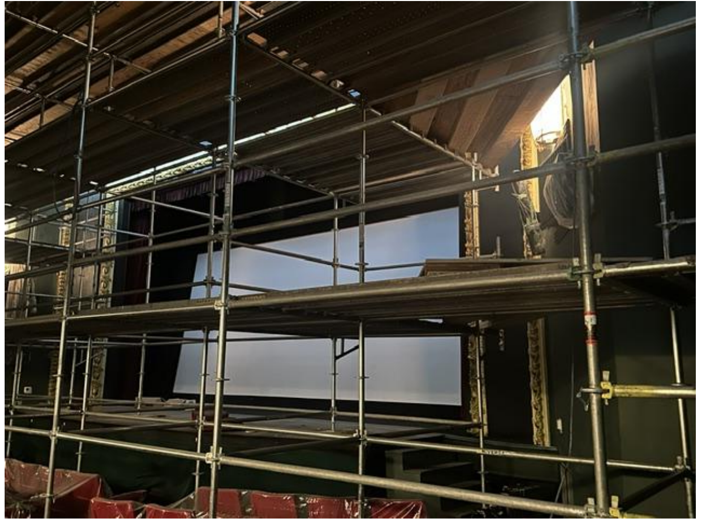
A view of the movie screen through the scaffolding installed throughout the Windsor Theatre auditorium in preparation for ceiling repairs
