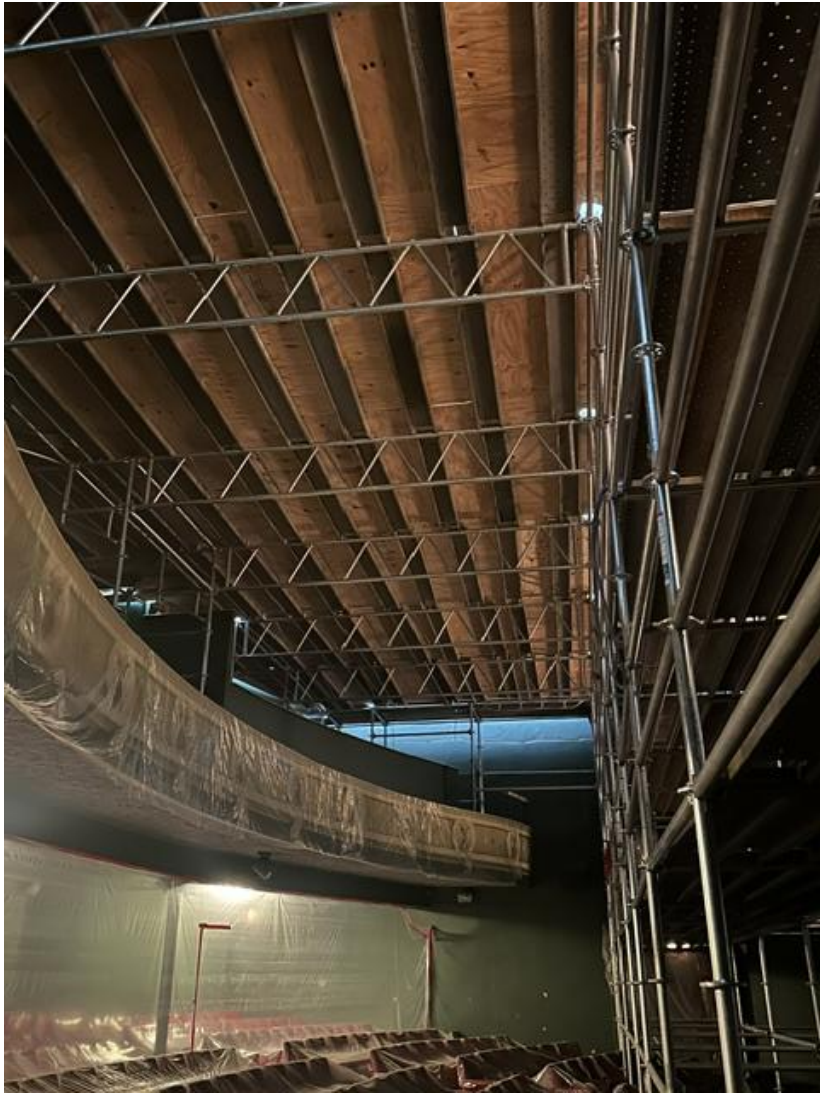
Plywood flooring has been installed on top of the scaffolding, providing a platform for workers to stand on while reaching the Windsor Theatre auditorium ceiling.
